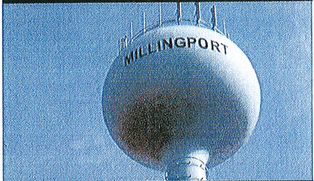
FIGURE 2. The Millingport tank is a 200,000 gallon pedisphere. Because of low demand, turn-over in this tank is low.
